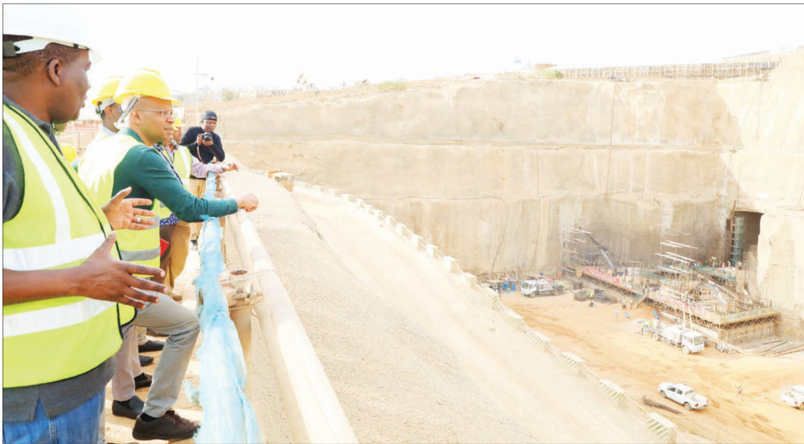
Energy minister January Makamba (2nd-L) has a first-hand account of progress in the implementation of the Julius Nyerere Hydropower Station project in Rufiji District, Coast Region, yesterday. Left is the project's resident engineer John Mageni. Photo: Correspondent Theresia Mhagama
