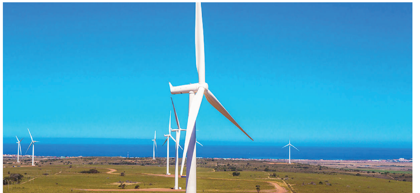
A wind farm at Jeffrey's Bay in the Eastern Cape.
