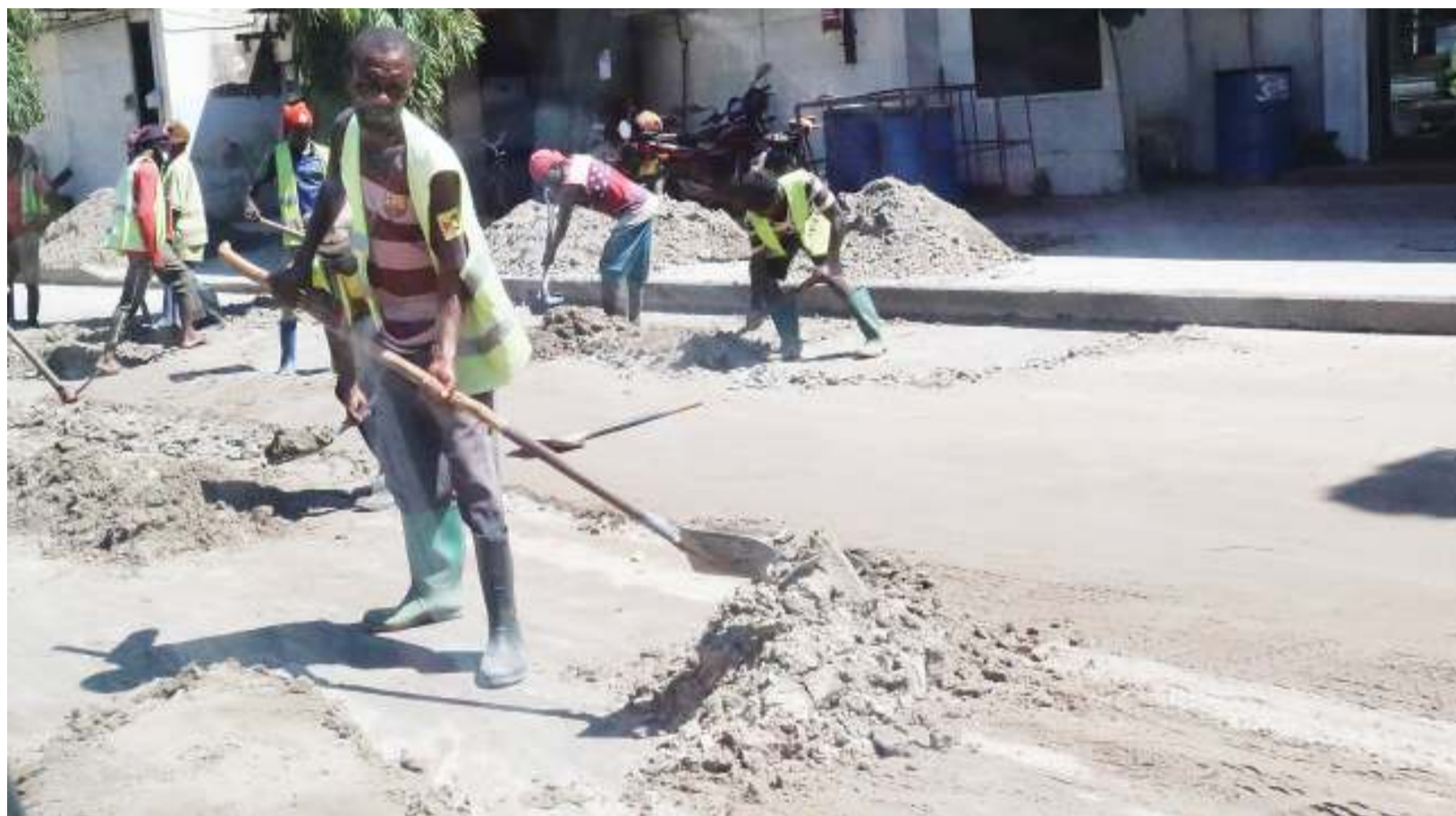
Casual workers removing sand from a wide range of road surface along Nyerere road at Gold Star area in Dar es Salaam yesterday. Photo: Selemani Mpochi
