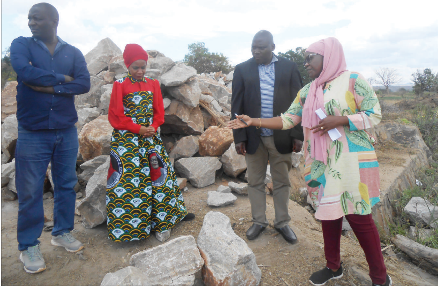
Zuhura Aman (R), head of Tanzania National Roads Agency's (Tanroads) road maintenance department for Tanga Region, briefs Kilindi district commissioner Abel Busalama (2nd-R) yesterday on the progress made in the construction of Songe bridge. Photo: Correspondent Dege Masoli
