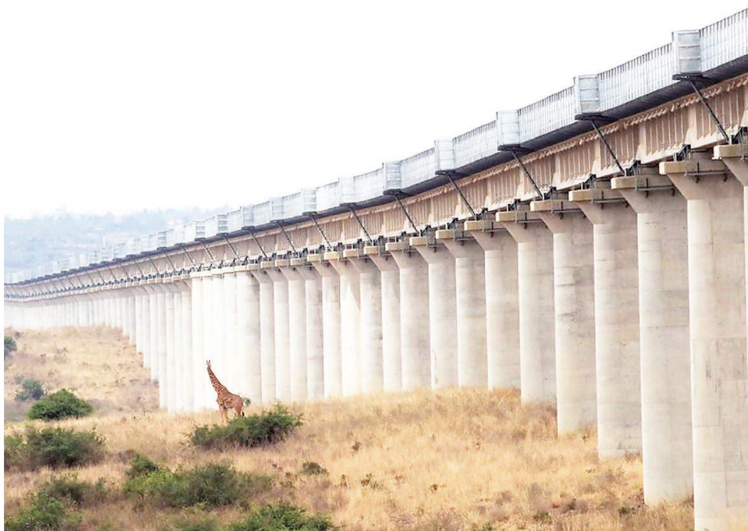
A giraffe walks near an elevated railway line that allows movement of animals below the Standard Gauge Railway line linking Nairobi and Naivasha, inside the Nairobi National Park.
