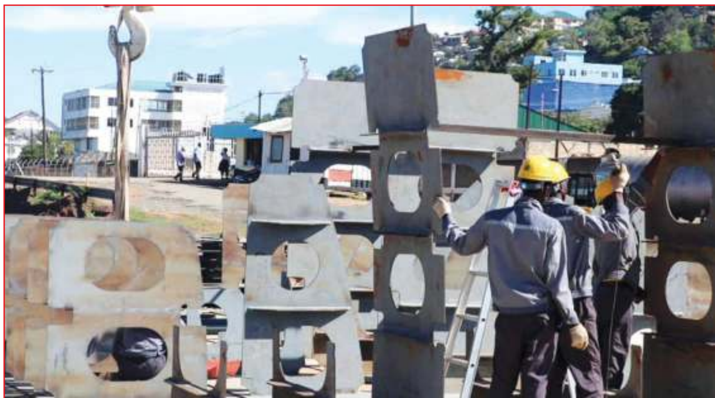
Assembling of steel blocks as part of new shipbuilding in progress at Mwanza South Port. The project of new shipbuilding which will be having a carrying capacity of 1,200 passengers and 400 tons upon its completion hence making it the biggest Passenger Cum Cargo vessel along Lake Victoria, is being implemented by GAS Entec Co. Ltd. in Joint Venture with Kang Nam Co. Ltd. (both from South Korea) and SUMA JKT. The new ship is expected to be ready for operations by the beginning of year 2021.
