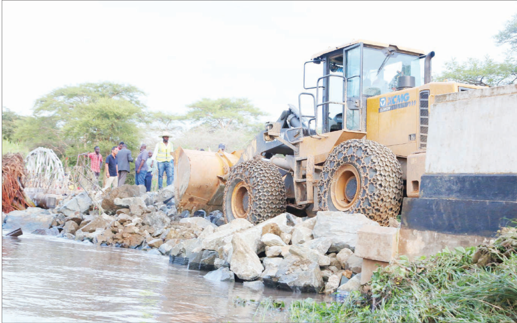
Graders are commonly used in the construction and maintenance of dirt roads and gravel roads. In the construction of paved roads, they are used to prepare the base course to create a wide flat surface upon which to place the road surface. A Grader at the rehabilitation of Lupa river bridge linking Chunya-Makongorosi in Mbeya which was swept away by floods recently. Photo: Correspondent Nebart Msokwa
