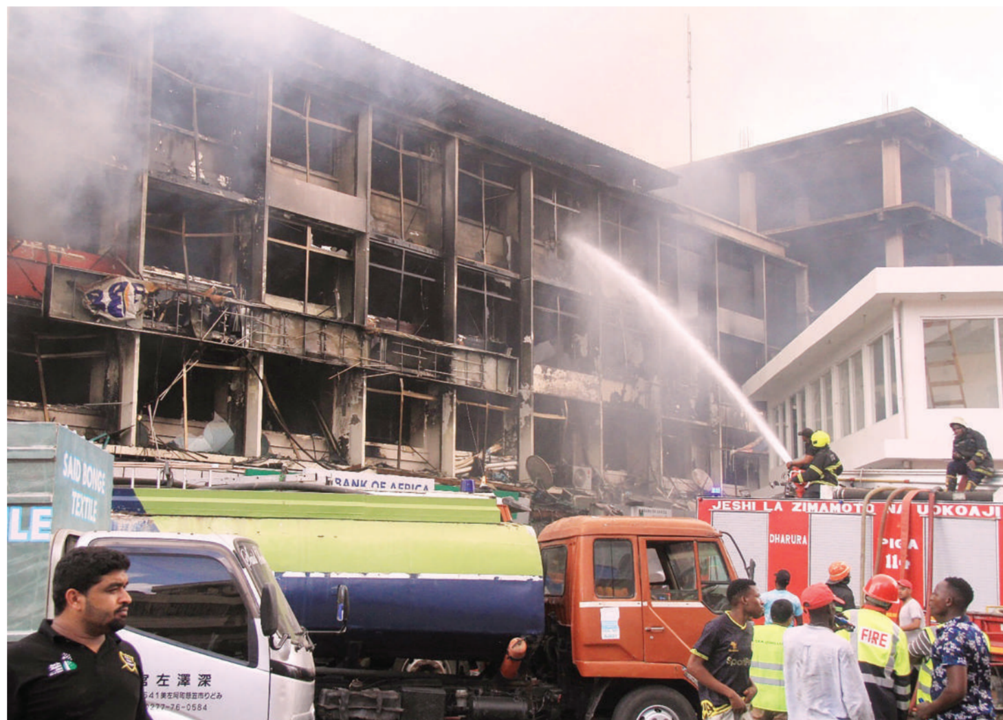
Fire and Rescue Force members pictured yesterday fighting to put out a morning fire which gutted several commercial and other buildings along Msimbazi Street in Dar es Salaam's sprawling Kariakoo Market zone. Photo: Correspondent Jumanne Juma
