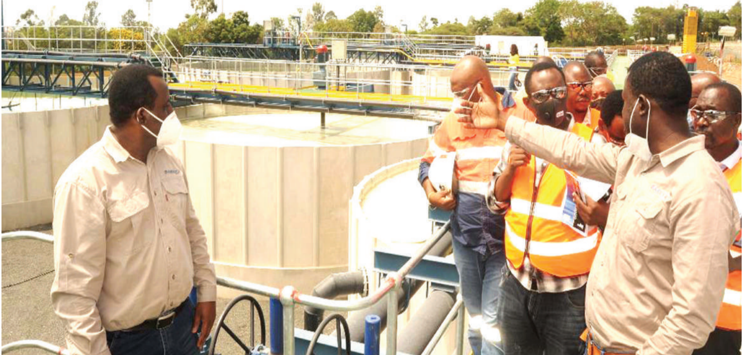
Barrick North Mara Gold Mine's process plant manager, Christopher Mwinuka (R) explains to journalists on how the new waste water treatment plant works at the mining site in Tarime mid earlier this week. Looking on (L) is the mine's general manager, Apolinary Lyambiko. Photo: John Badi.
