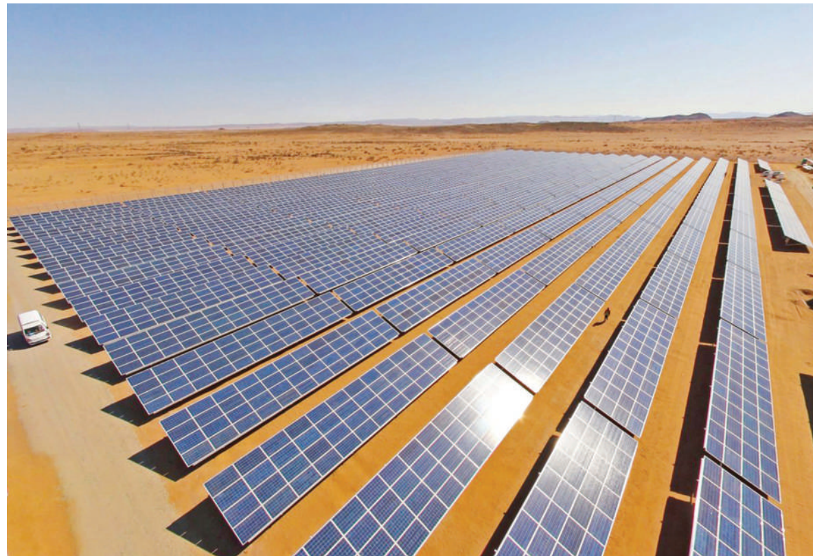
The electricity will be supplied to five Tronox facilities in the Western Cape and KwaZulu-Natal
