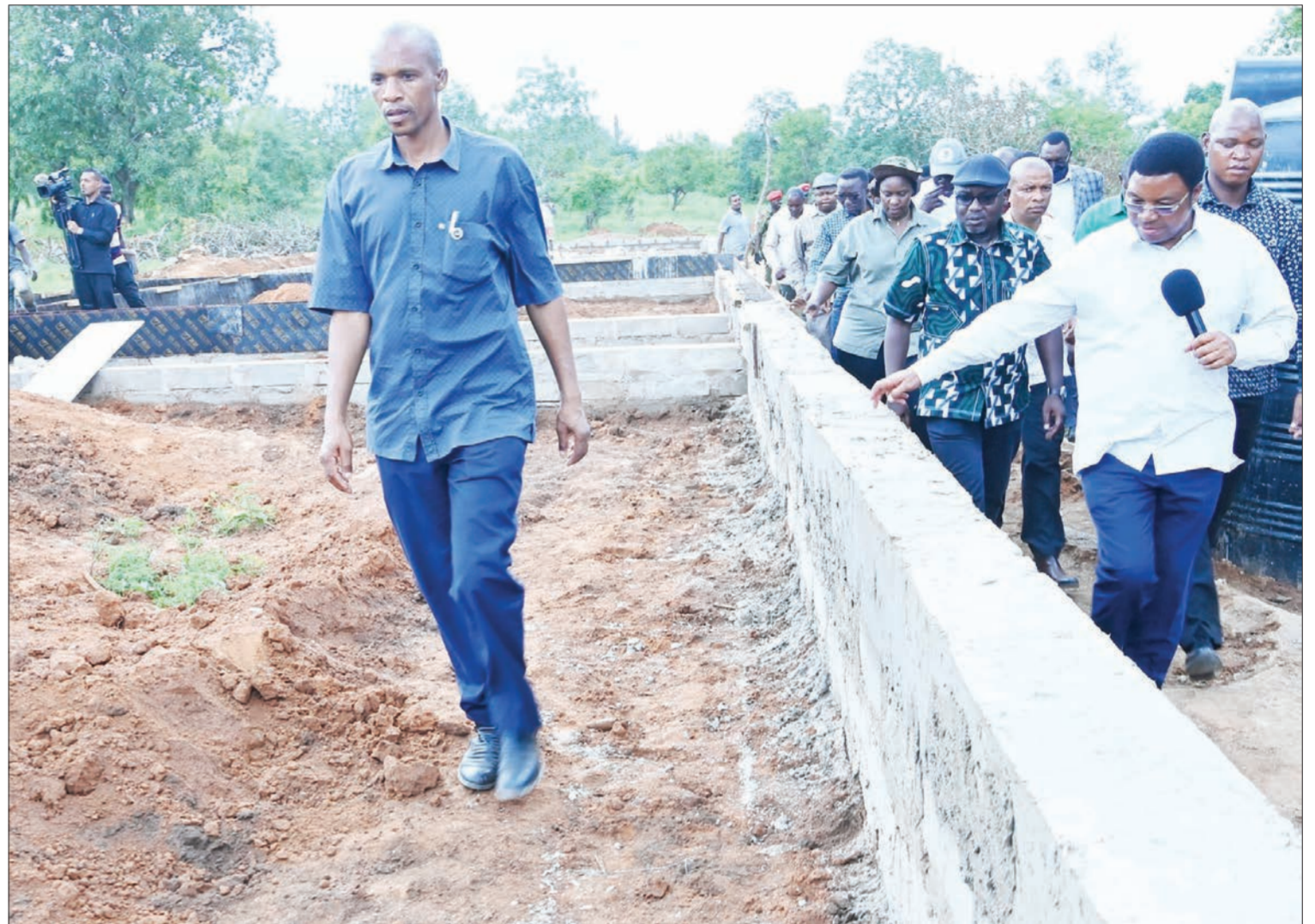
Prime Minister Kassim Majaliwa (R, with microphone) pictured yesterday having a first-hand account of the construction of primary school classrooms at Msomera in Handeni District. The facilities are meant for people set to move from Ngorongoro Conservation Area for resettlement in the village. Photo: PMO
