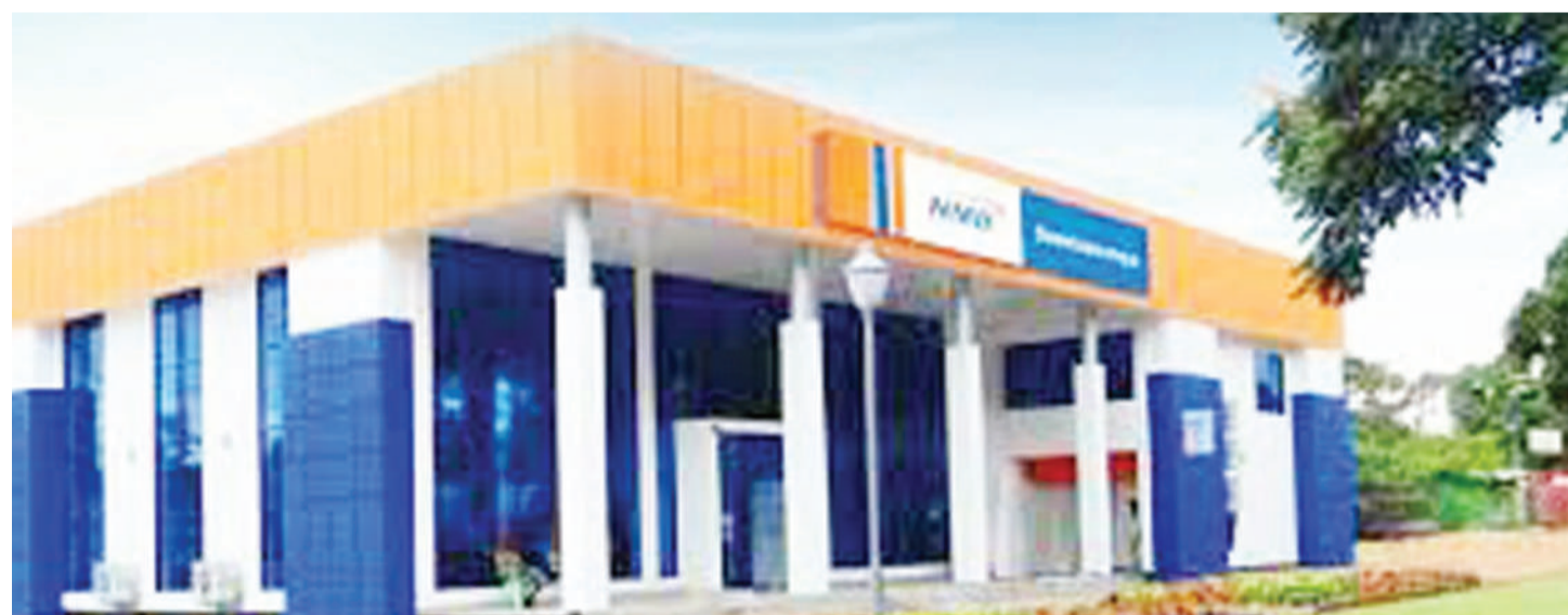
NMB Bank main branch in Zanzibar.
