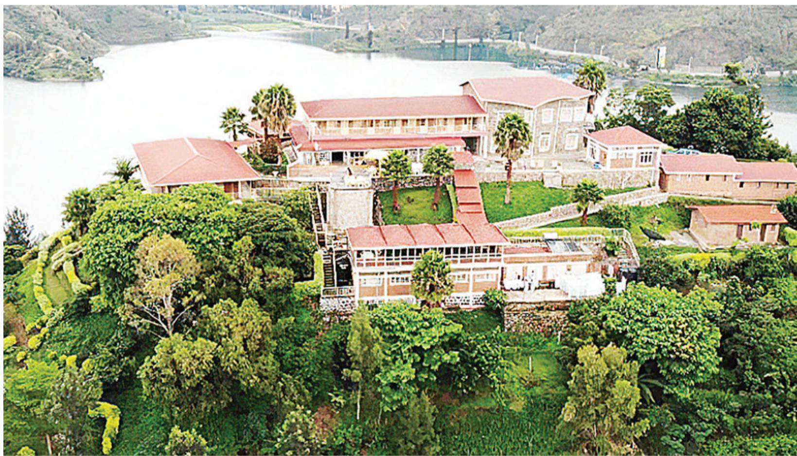
An aerial view of Saint Jean Hotel in Karongi District on the shores of Lake Kivu.
