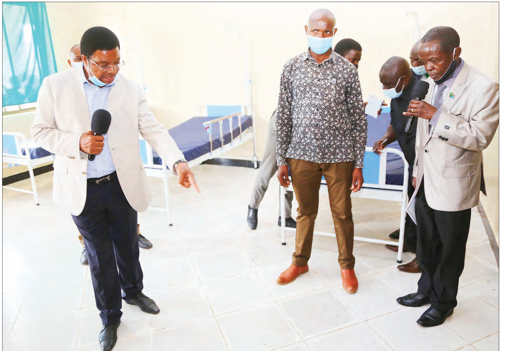
Prime Minister Kassim Majaliwa, who is on a tour of Kagera Region, pictured yesterday ordering that tiles used in the construction of Karagwe District Hospital's maternity ward floor be removed and replaced. This followed confirmation that they were of substandard quality. Photo: PMO
