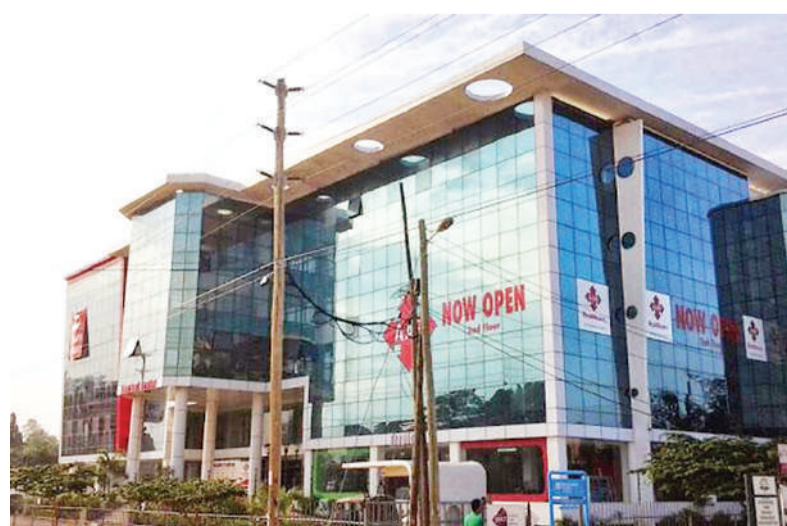
AAR head offices in Dar es Salaam.
