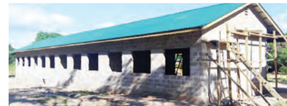
LEADERS ARRESTED OVER FAILURE TO SUPERVISE CLASSROOM BUILDING PAGE 6
