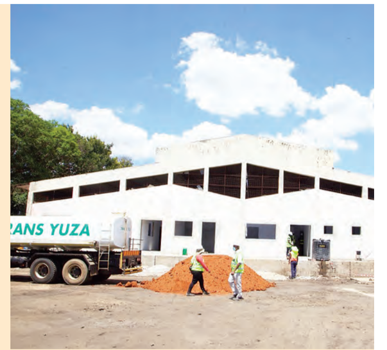
Construction of the dry port under way in Ressano Garcia.
