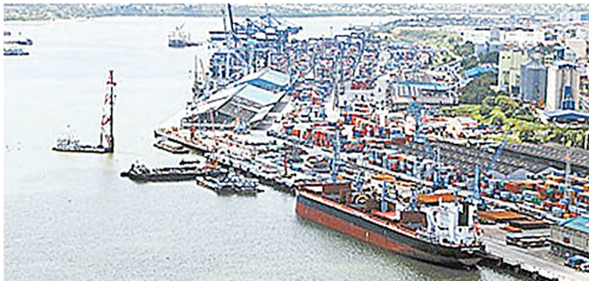
An aerial view of Dar es Salaam Port which incorporates an electrical workshop.
