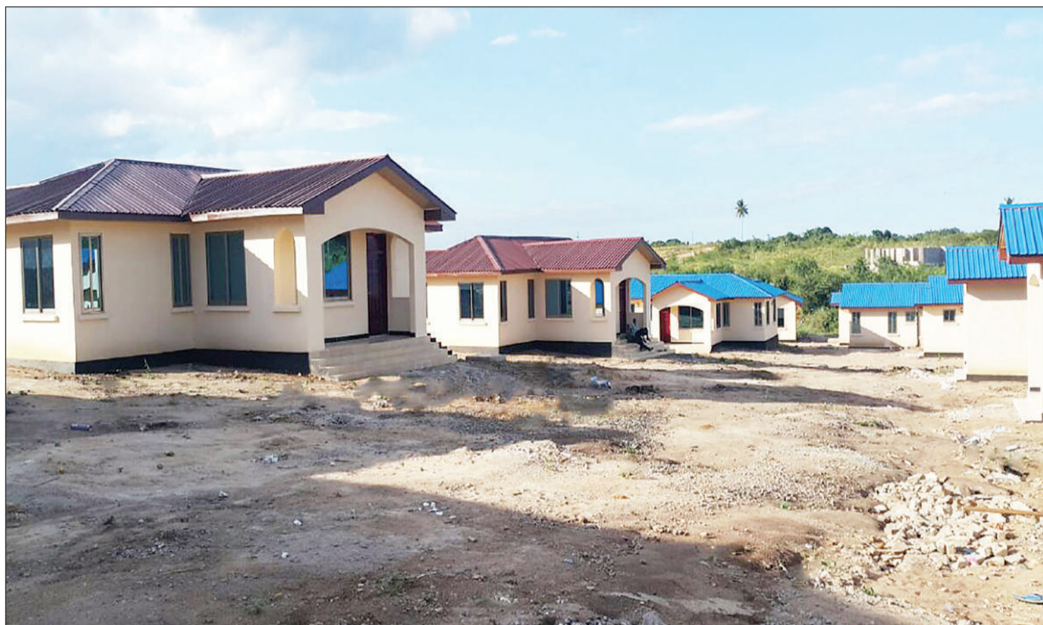
WHC's Gezaulole houses in Dar es Salaam.
