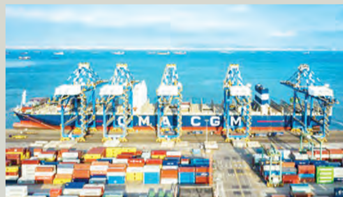
A vessel is docked at a container terminal of the Guangzhou Port, Nansha District, Guangzhou, south China's Guangdong Province, Feb. 13. File Photo
