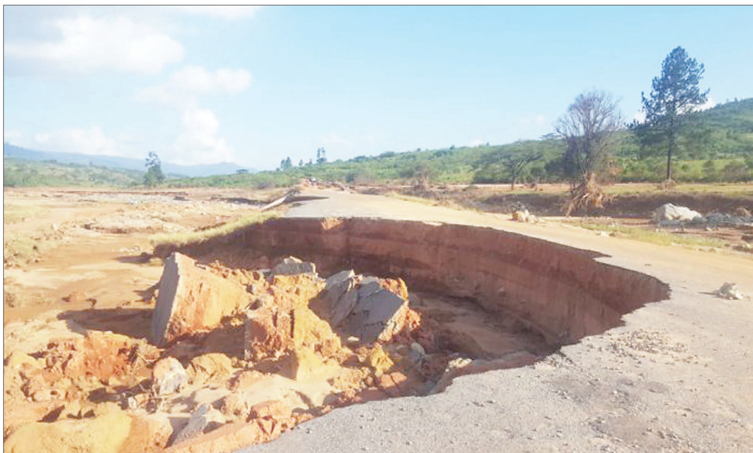
Cyclone Idai left a trail of destruction in Zimbabwe's Chimanimani district, in March 2019.
