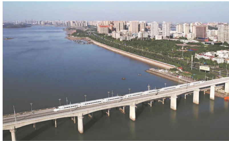
A high-speed train crosses a bridge of the Fangchenggang-Dongxing Railway in the Guangxi Zhuang autonomous region.
