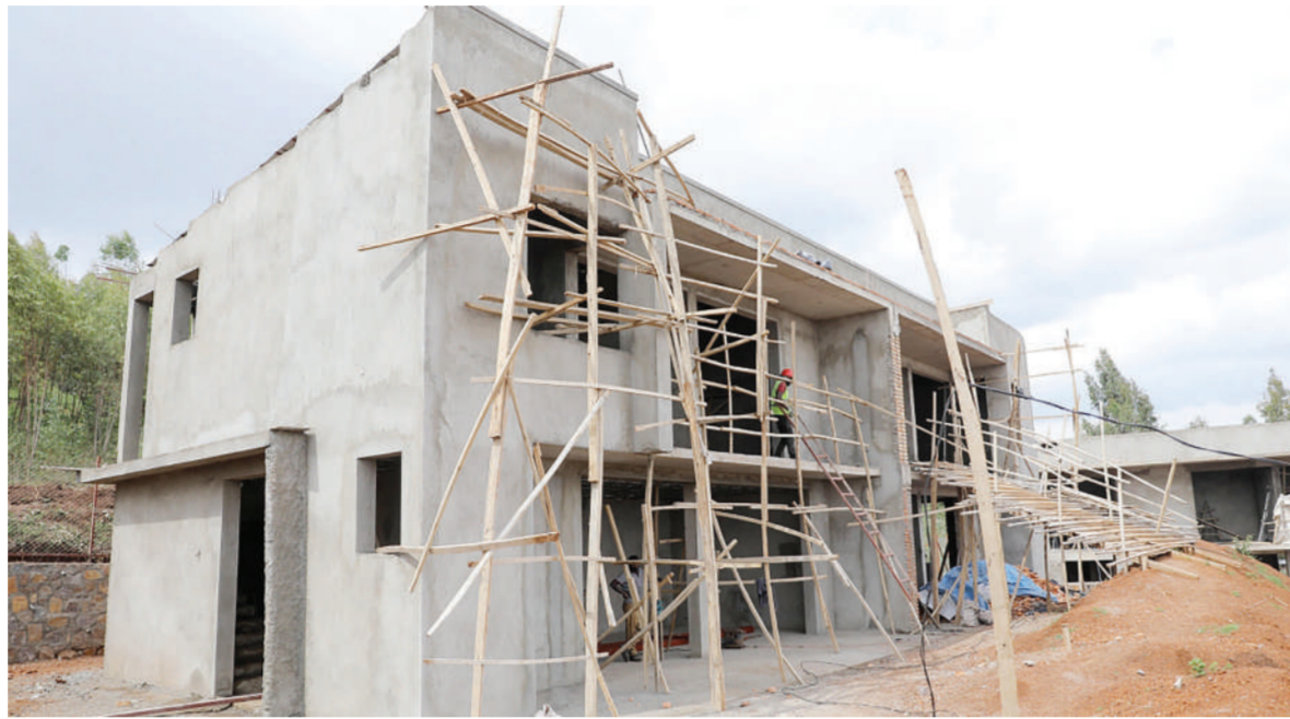
A construction site.
