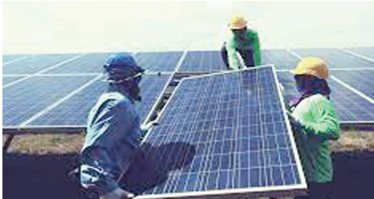
Workers install solar panels at a power plant in Maroua, Cameroon.
