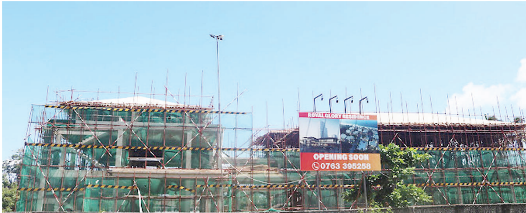
Stalled Royal Glory Residence project in Mikocheni, Dar es Salaam
