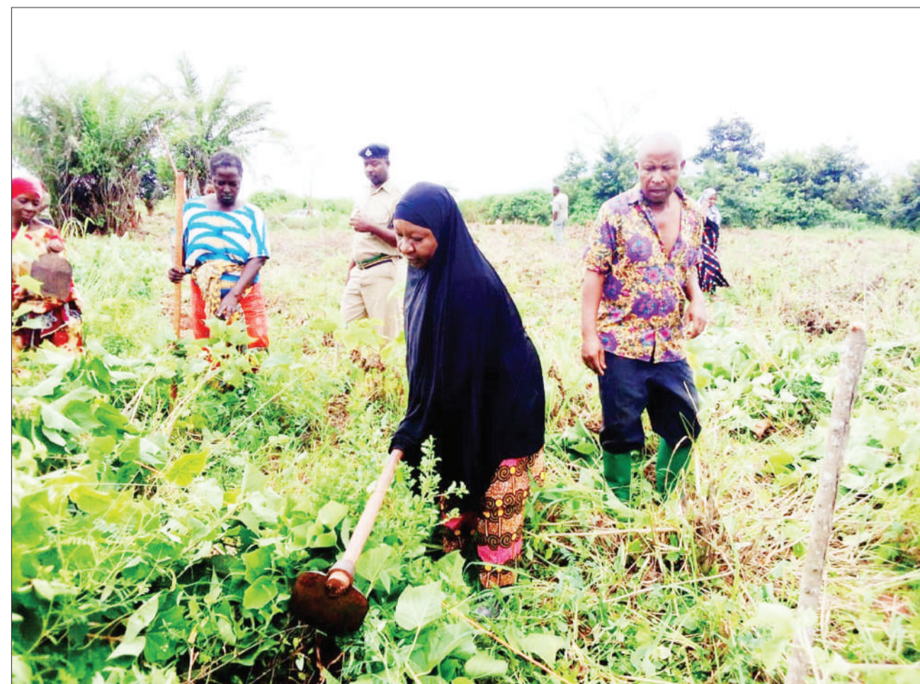
Mueha district commissioner Mwanasha Tumbo (with hoe) pictured on Wednesday taking part in clearing a site at Upare village that is earmarked for the construction of a dispensary. Photo: Correspondent Steve William
