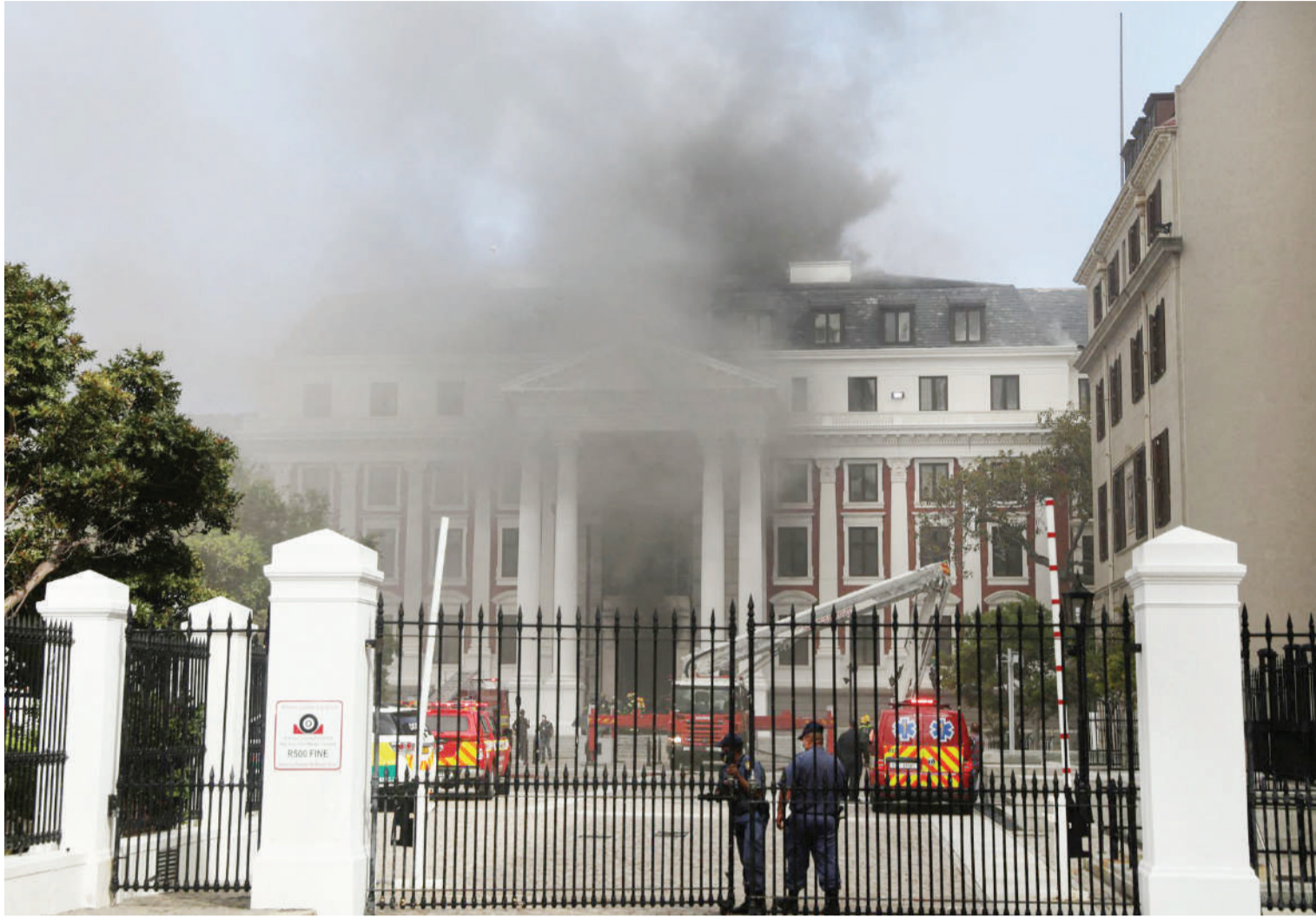
Parliament in Cape Town burns on 3 January 2022. The damage has not been repaired, although money has been made available, and much of MPs' work continues to be done in virtual settings. (Photo: ER Lombard / Gallo Images)
