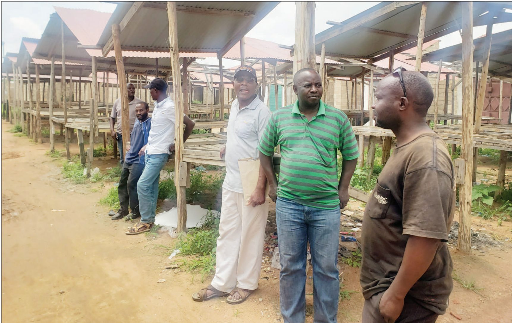
Residents of Nkhungu ward in Dodoma Urban District look on forlornly at structures that were meant for use as a mixed-goods market but have stood unused since they were ready for business some nine years ago, with traders reportedly opting for unauthorised sites. Photo: Correspondent Paul Mabeja
