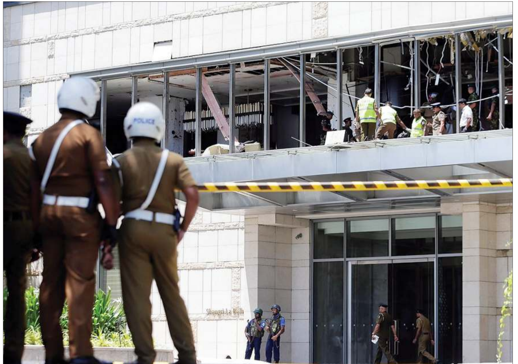
Police and forensic officials inspect the site of an explosion at the Shangri-la hotel in Colombo, Sri Lanka, on April 21, 2019. AP Photo
