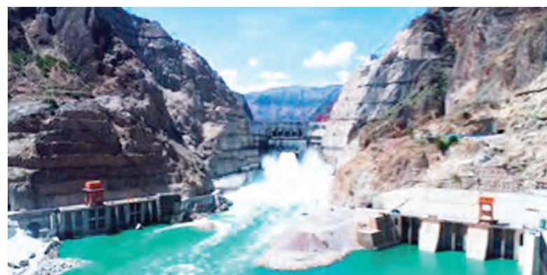
An overview of Wudongde hydropower plant
