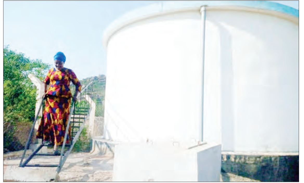
Taabu Machumu, special seats councillor for Makojo ward in Musoma Rural constituency, inspects a Lake Victoria water project being implemented by the National Water Fund and meant to benefit Makojo and Chitare villages. Photo: Guardian Correspondent
