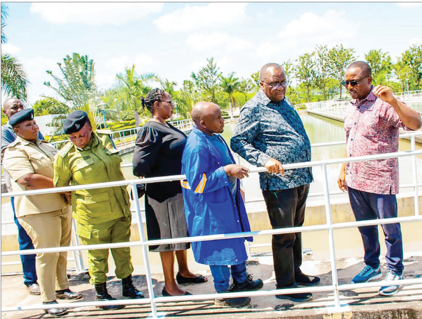
Shinyanga regional Water Supply and Sewerage Authority director Patrick Nzamba (R) pictured yesterday taking a delegation led by Shinyanga regional commissioner Anamringi Macha (2nd-R) around a project meant to distribute Lake Victoria water pumped from Ihelele in Misungwi District in Mwanza Region. Photo: Guardian Correspondent
