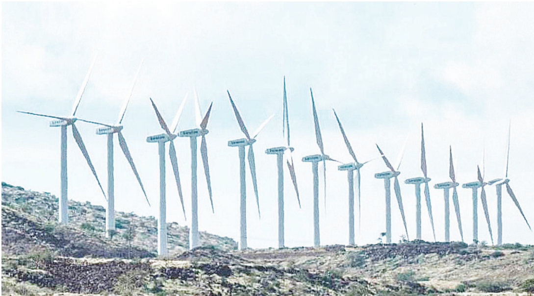
Wind turbines at the Lake Turkana Wind Power project.
