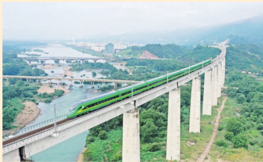
A bullet train runs on a bridge of Jinhua-Taizhou railway in east China's Zhejiang province, June 18, 2021. The train can run as much as 160 kilometers per hour. (Photo by Wang Huabin/People's Daily Online)
