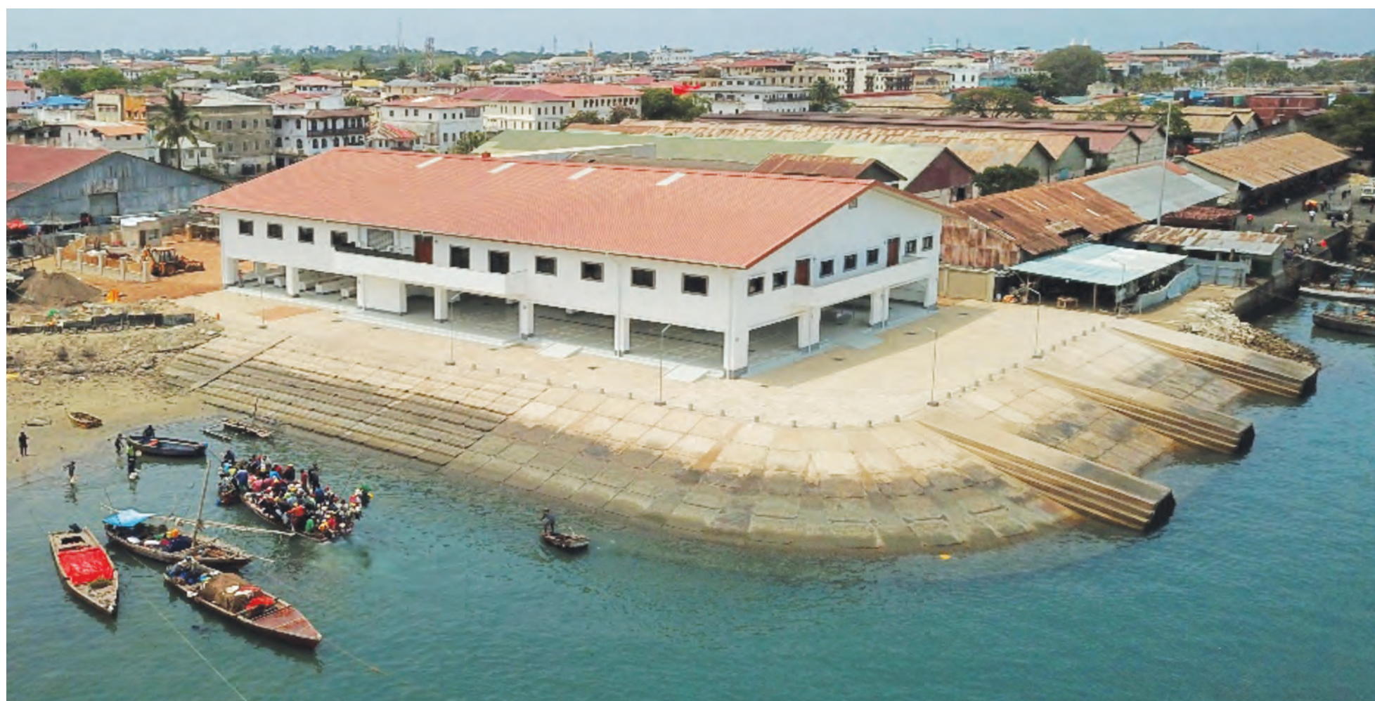
New Malindi fish landing and marketing facilities. Clean and safety.
