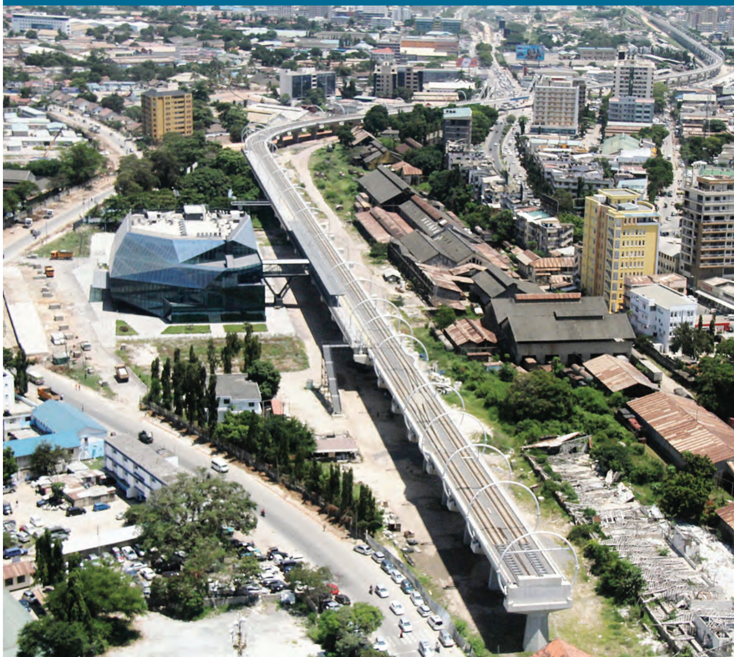
AN aerial view of a section of the completed Dar es Salaam-Morogoro stretch of the Standard Gauge Railway, as captured yesterday. Photo: Correspondent Jumanne Juma
