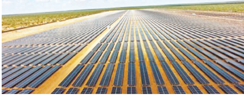
The 50 MW Garissa Solar Power Plant, consisting of over 200,000 photovoltaic panels, covers an area of 85 hectares. It is by far the largest photovoltaic power project in Kenya, and even in East Africa.
