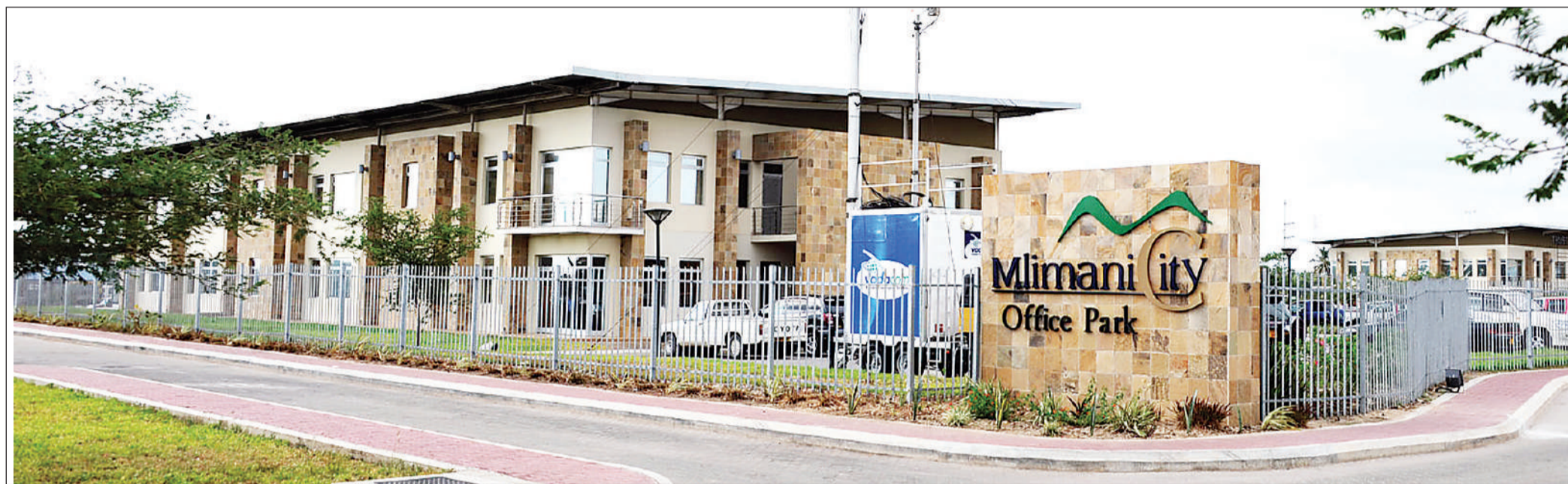
An office block at Dar es Salaam Mlimani City office park
