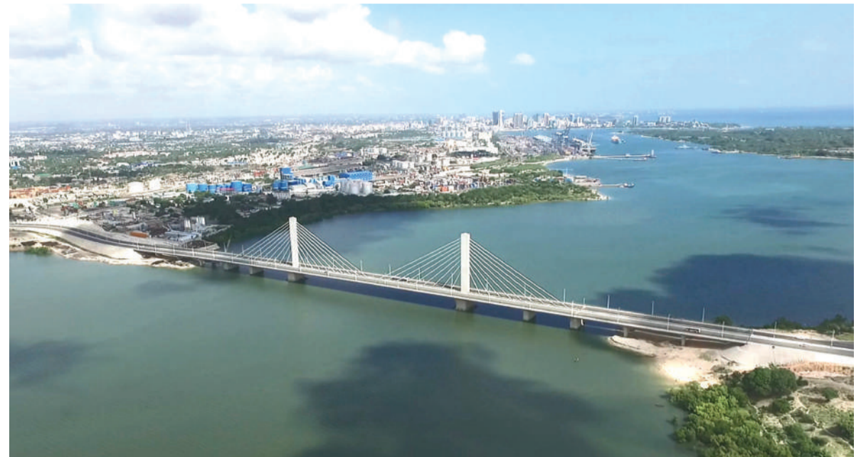
The Nyerere Bridge in Dar es Salaam was built by a Chinese company from Sept. 2012 to April 2016. It is the first cable-stayed, sea-crossing bridge in East Africa. (Photo/CRJE)
