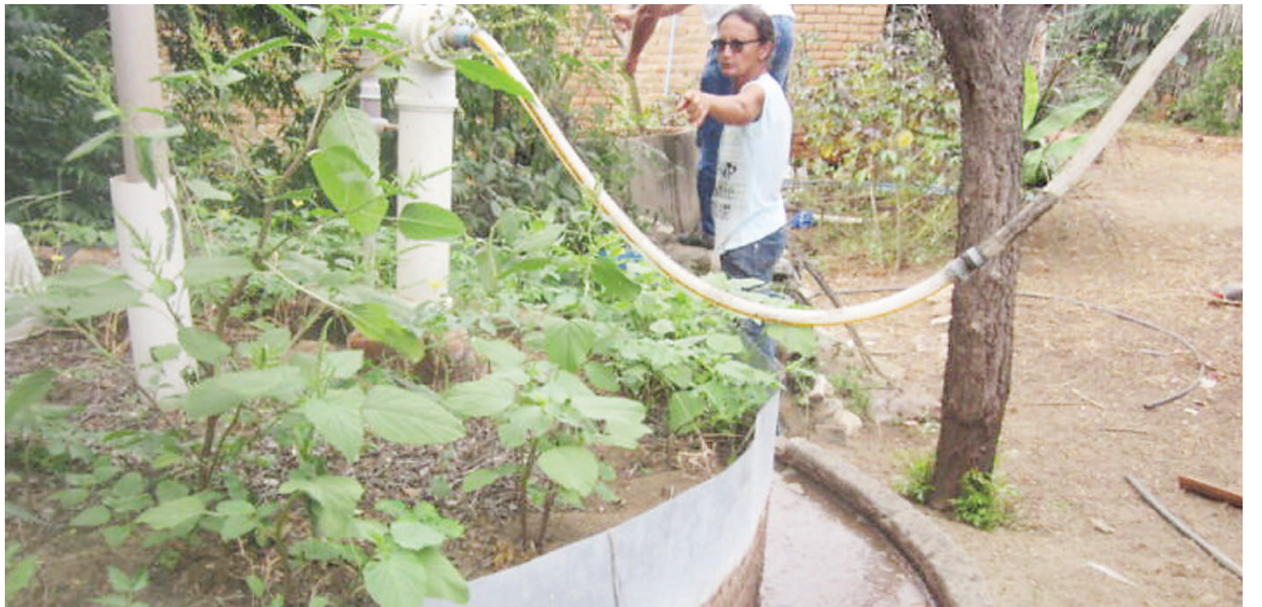
Farmer Maria das Dores Alves da Silva stands between the manure pit and the “sertanejo” biodigester designed by Diaconia, a social organization of Protestant churches in Brazil, which has already installed 713 biogas production plants in eight of Brazil’s 26 states. CREDIT: Mario Osava / IPS
