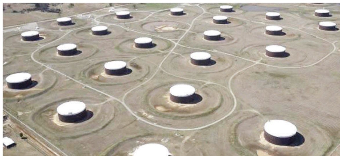
Crude oil storage tanks are seen from above at the Cushing oil hub in Cushing
