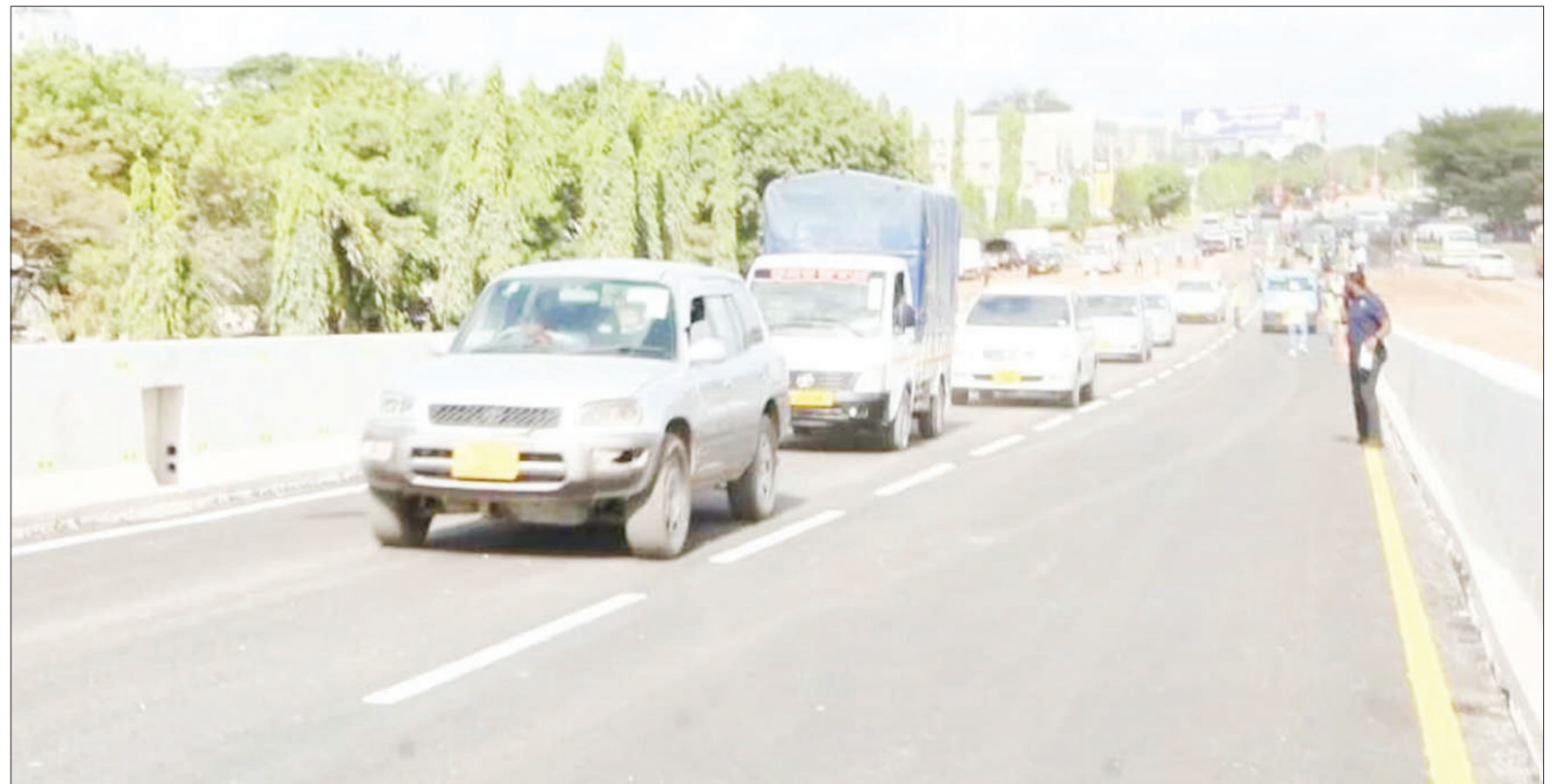
Motor vehicles at Chang'ombe flyover along Nyerere Road in Dar es Salaam following the launch on Sunday by Works and Transport minister Prof Makame Mbarawa. Photo: Guardian Correspondent
