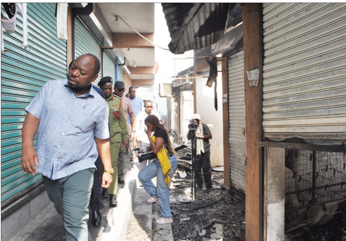
Albert Chalamila, the Dar es Salaam regional commissioner, inspects kiosks destroyed by fire at Mwenge area in Dar es Salaam yesterday. Photo: Correspondent Imani Nathaniel
