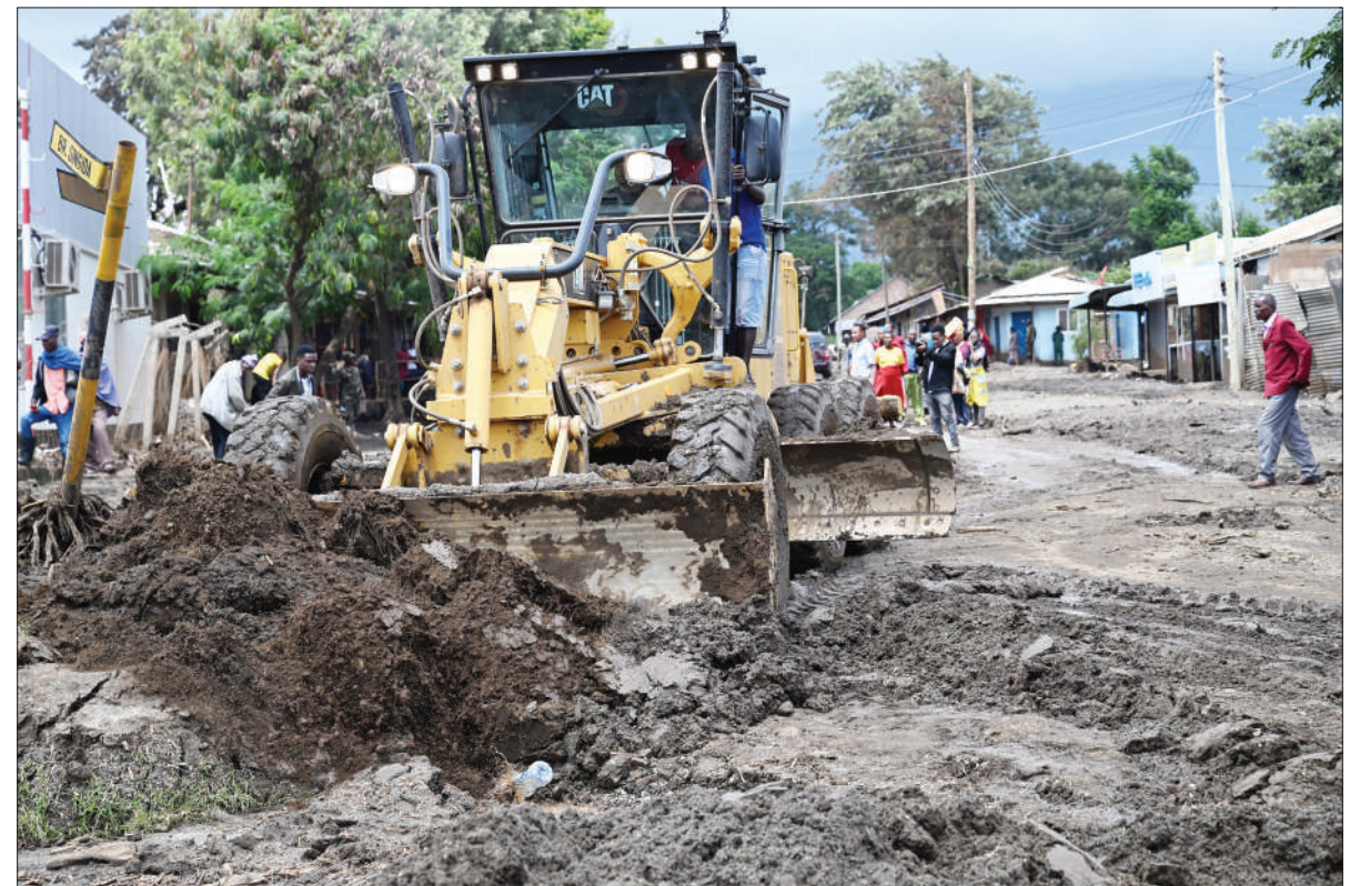
Grader removes mud scattered at Katesh bus stand following the mudflow caused by heavy rains occurring on Sunday. Photo: PMO
