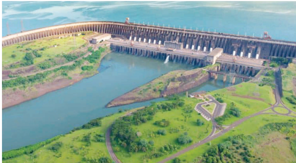
Mphanda Nkuwa hydroelectric dam
