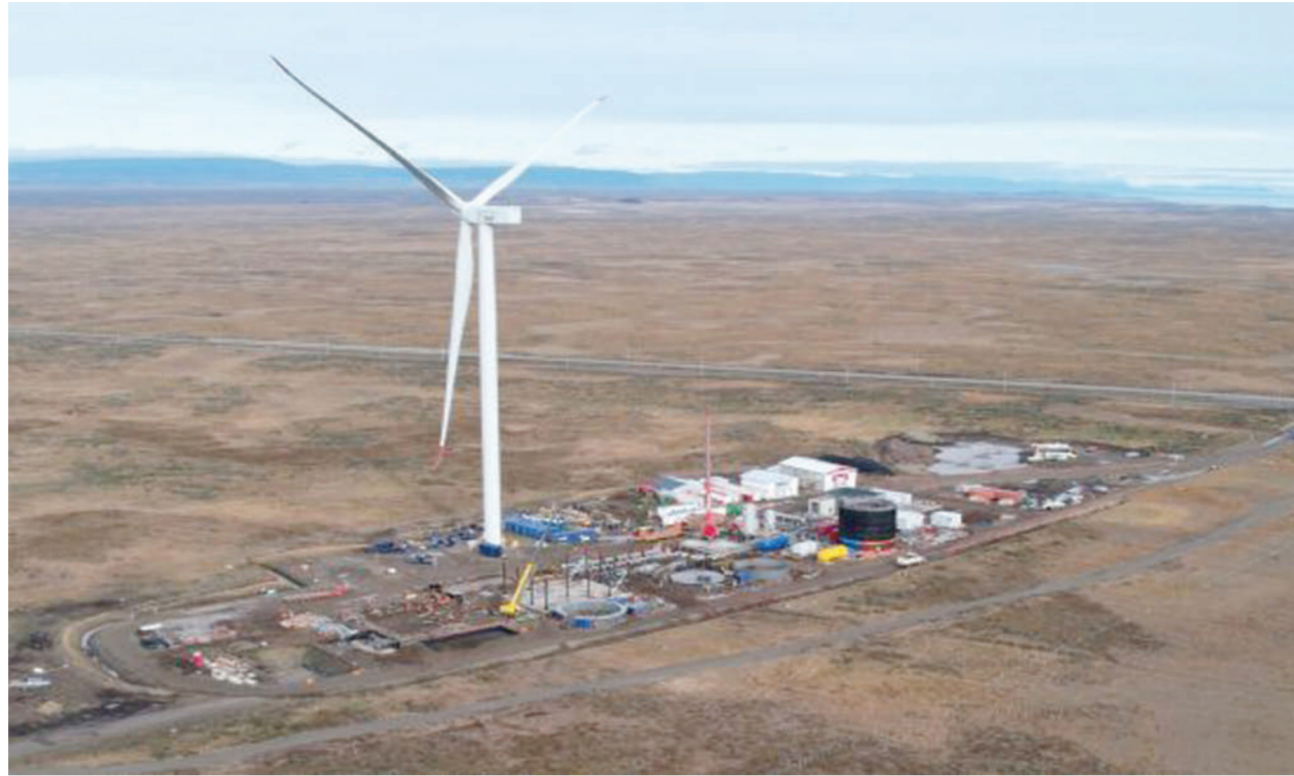
At the Haru Oni demonstration plant where the ecological fuel based on green hydrogen will be produced, the wind turbine that will provide wind energy to the project promoted by the HIF Global group in the southern Chilean region of Magallanes has been installed. CREDIT: HIF Global
