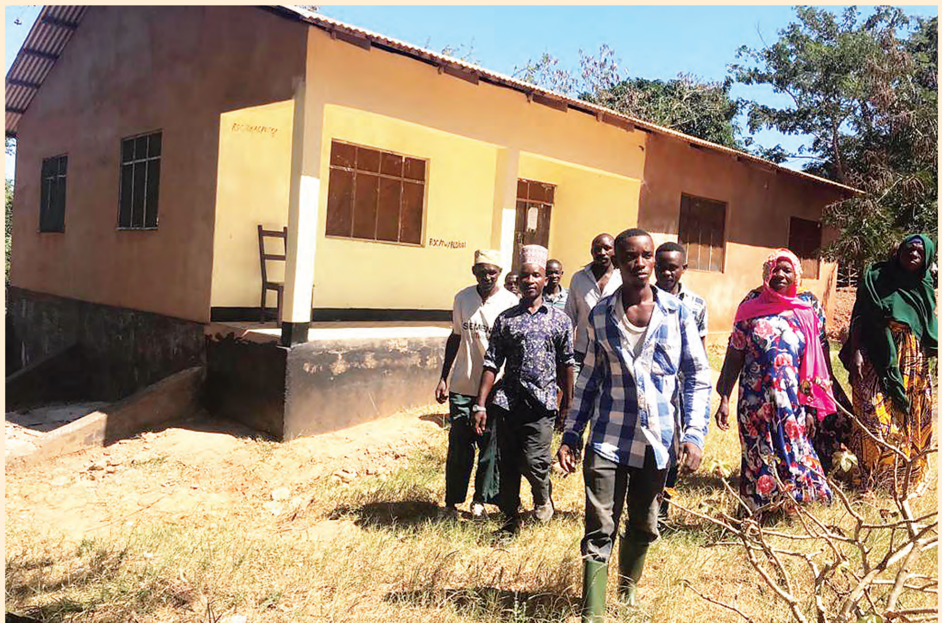
Tawi villagers in Rufiji district show the village office rehabilitated by the revenue accrued from CBFM. Photo: Correspondent Gerald Kitabu
