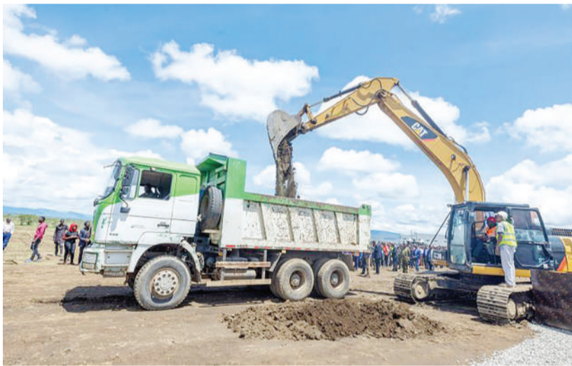
Groundbreaking ceremony for Raxio data centre. Photo Courtesy of Raxio group
