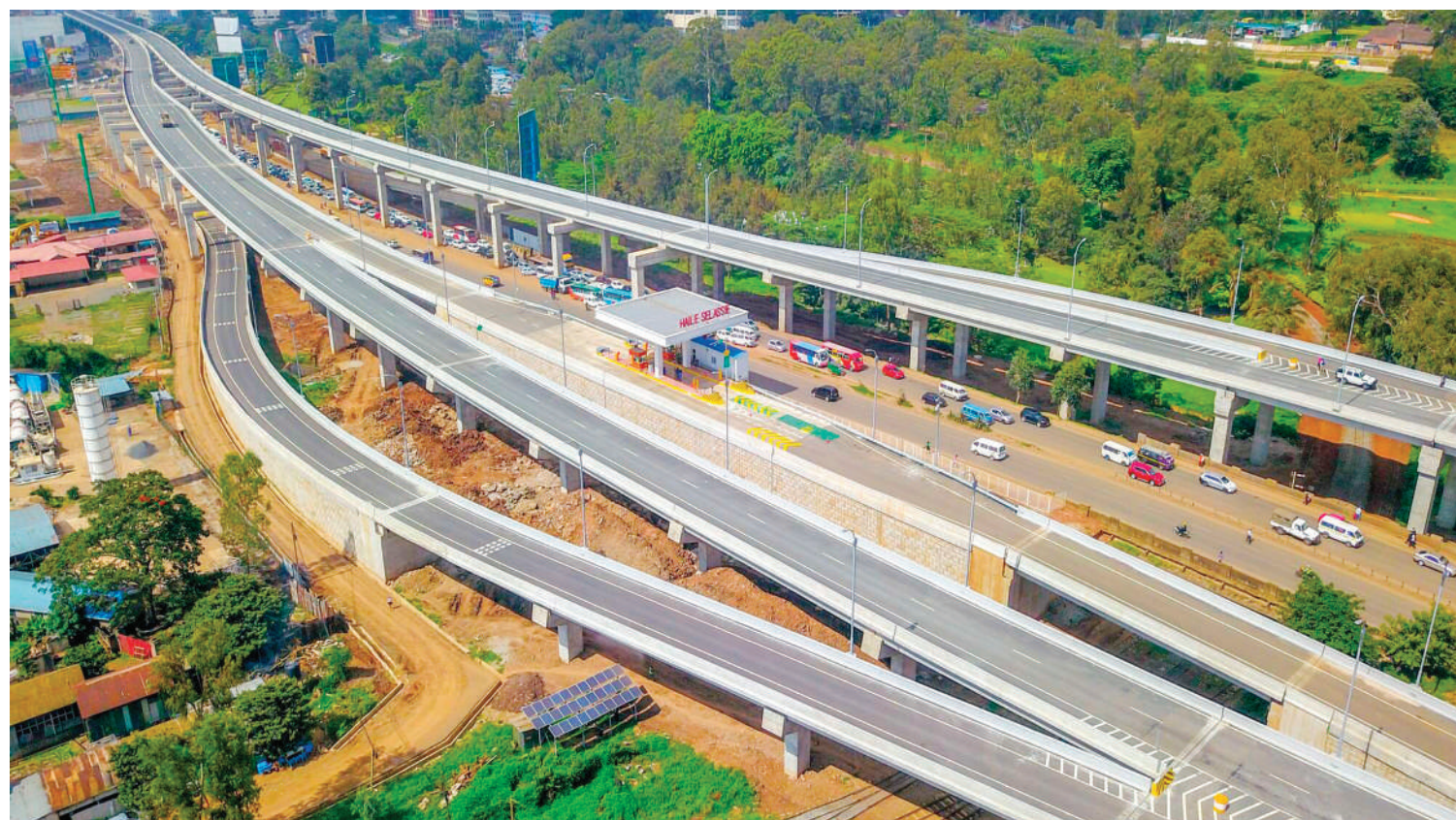
Part of the 27 km Nairobi Expressway
