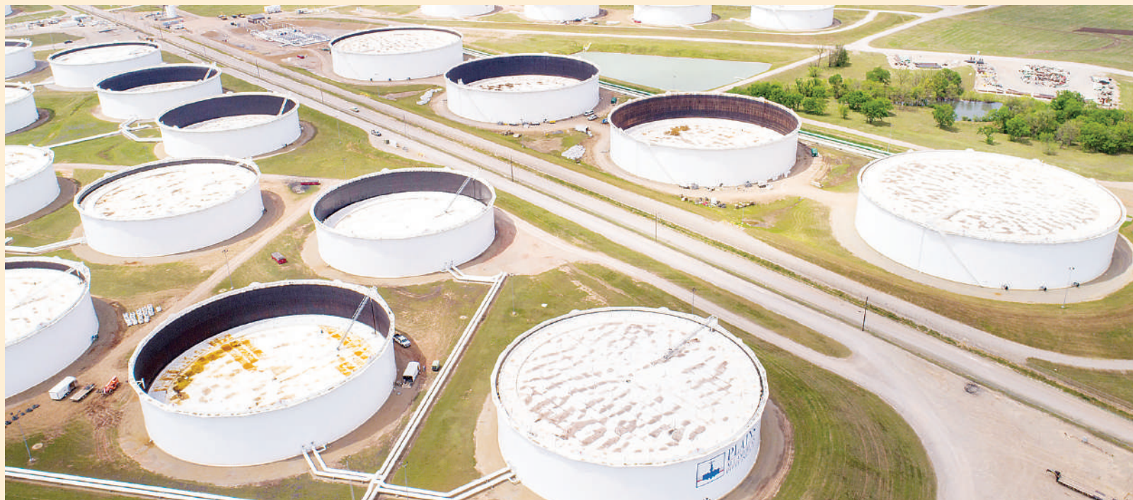
Oil storage facility
