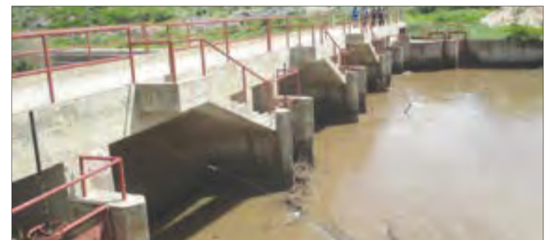
Construction of overhead irrigation facility.
