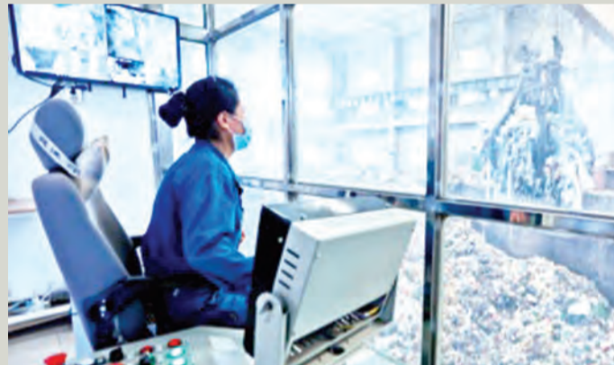
Photo taken on June 25, 2021 shows an employee of a biomass power generation company based in Zhangye, northwest China's Gansu province, operating grab bucket crane to move waste into receiving hopper.
