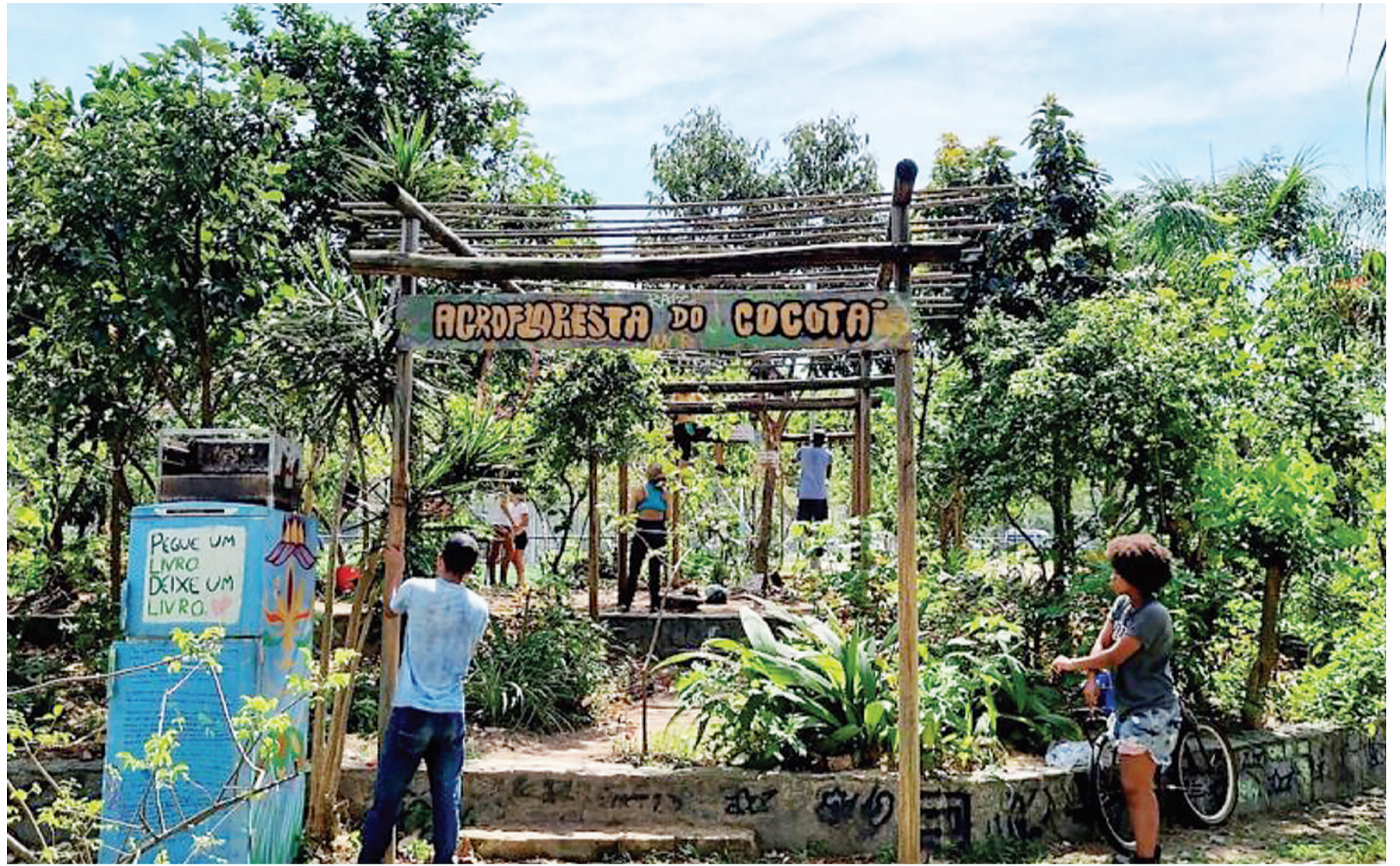
Building a pergola at the entrance to the Cocotá Agro-forest in 2023
