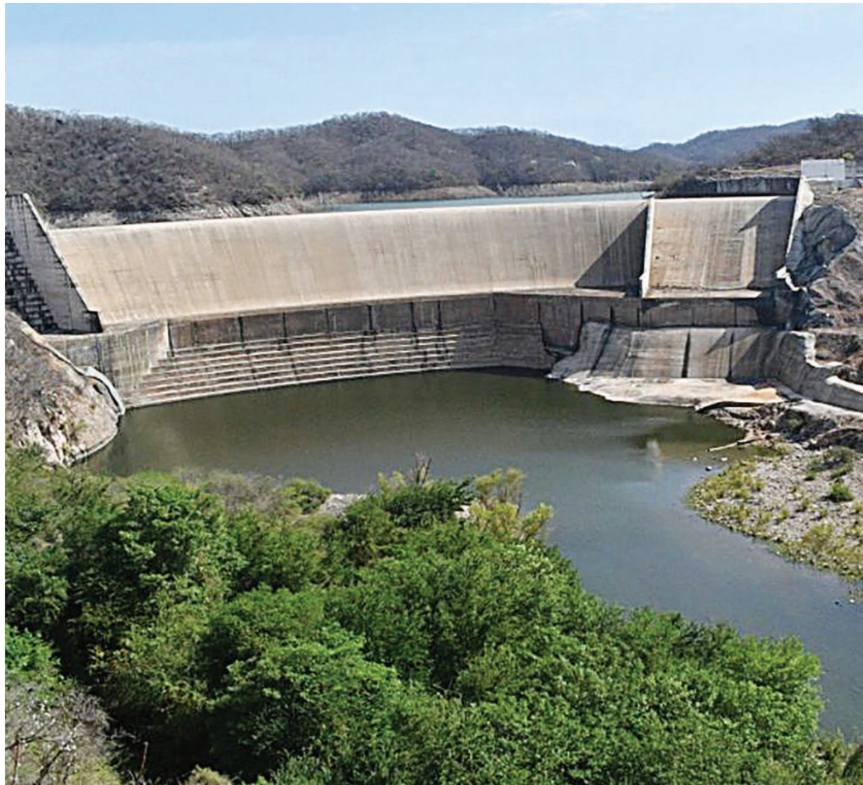
With a storage capacity of 580 million cubic meters and an irrigation target of 22,500 hectares, the Picachos dam in the state of Sinaloa, in northwestern Mexico, will also generate 15 megawatts of electricity. CREDIT: Conagua
