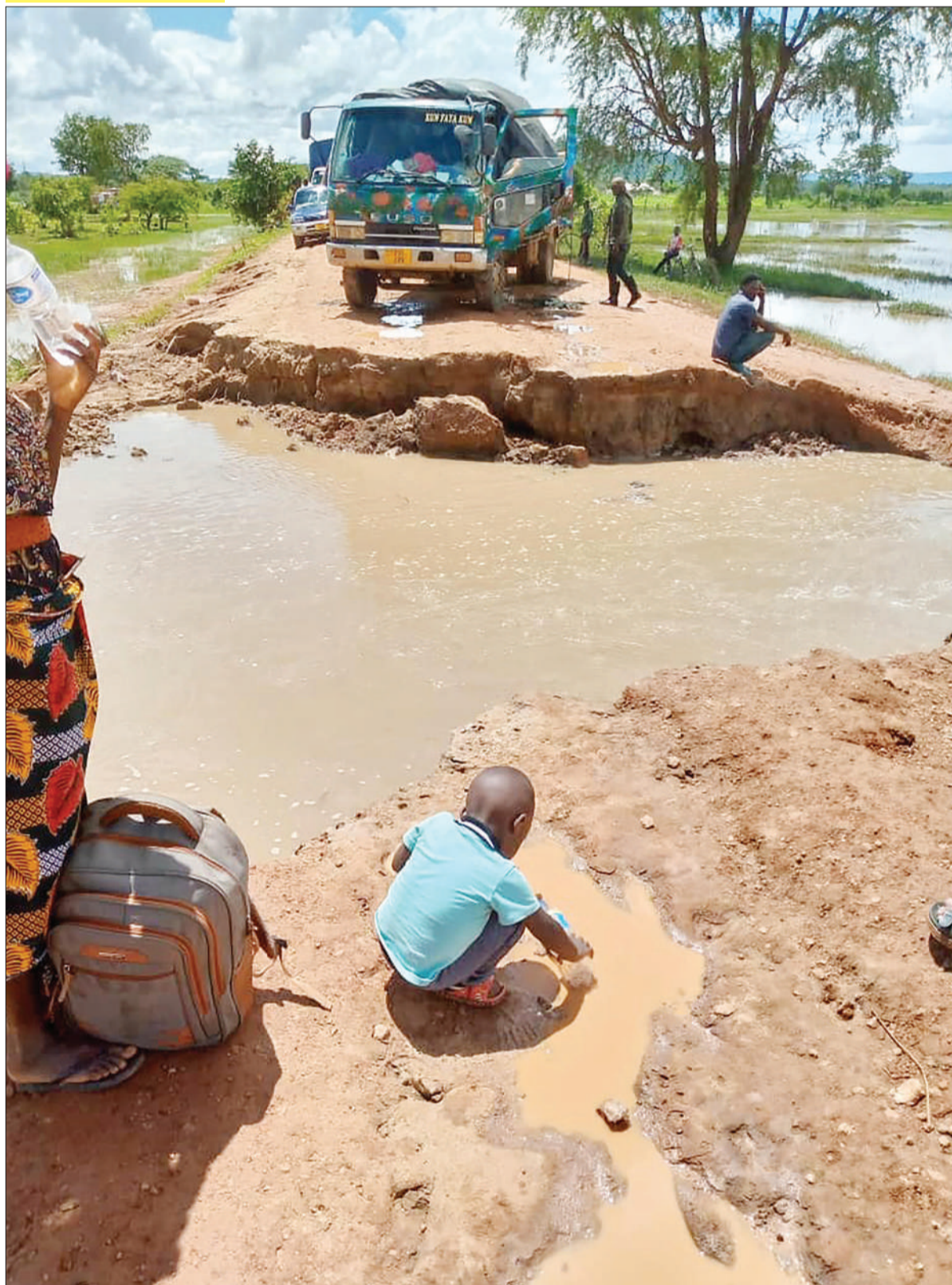
Ongoing rains have rendered this Kona ya Mnyagara section of a strategic road in Tanganyika District, Rukwa Region, impassable. Photo: Guardian Correspondent
